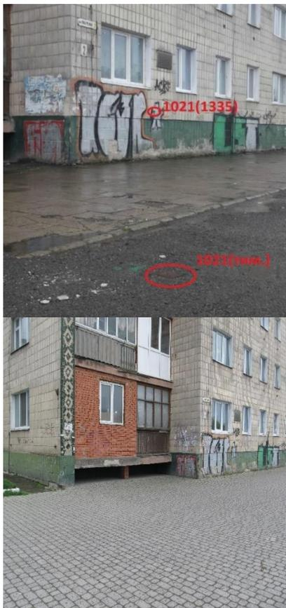
*Fig.2 "Closure" of the working center of the polygonal point by the pavement*
