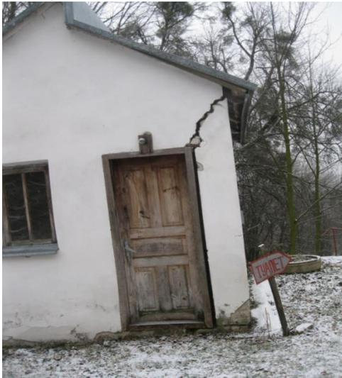
*Fig. 2. Photofixation of the crack (deformation) of the building on the territory of Podgoretsky monastery*
