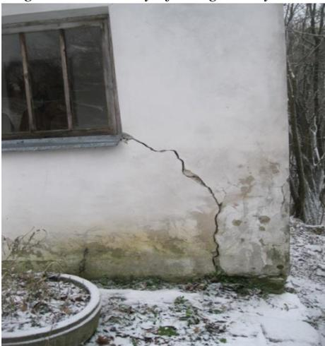
*Fig. 3. Photofixation of the crack (deformation) of the building on the territory of Podgoretsky monastery*
