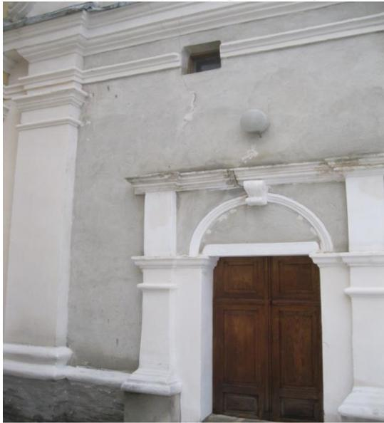
Fig. 6. Photofixation of the external fracture (deformation) above the entrance to the temple
