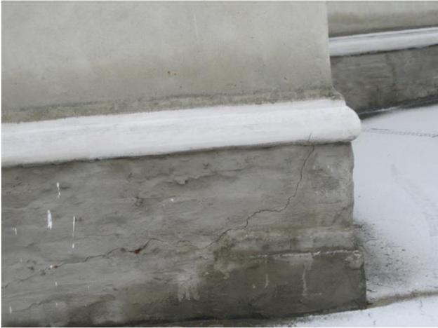
Fig. 5. Photofixation of the crack (deformation) of the foundation of the temple building
