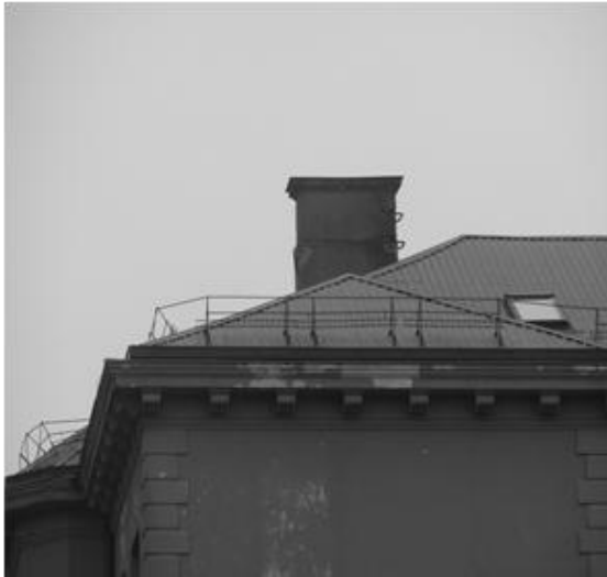
Fig.9. LatPos antenna installation location (Valka gymnasium)
